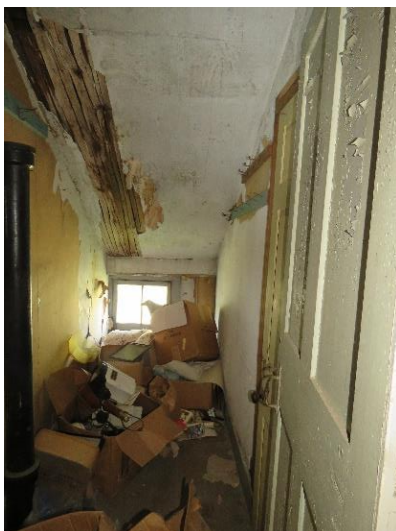
Figure 30 Ell Second Floor Door
