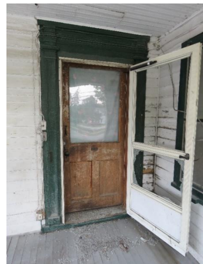
Figure 23 South Entry to Main Building
