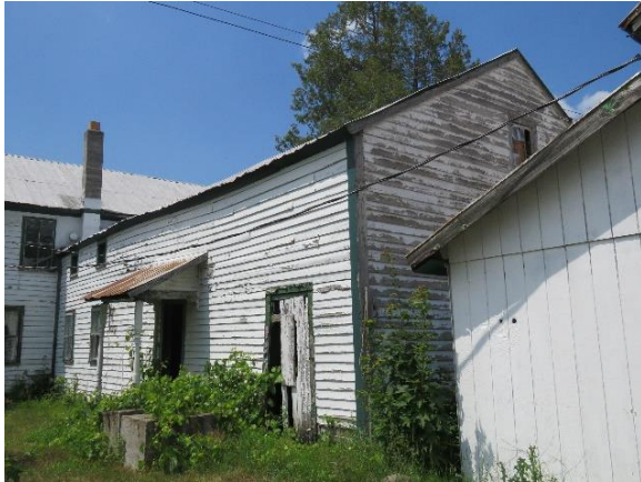
Figure 6 Ell Looking Northwest
