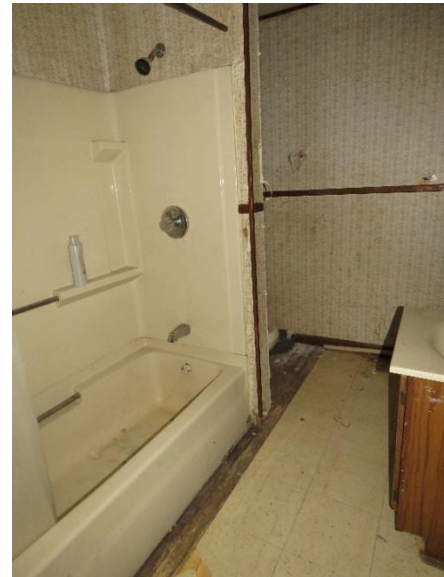
Figure 41 Main Building First Floor Bathroom
