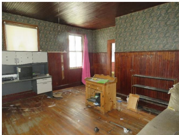
Figure 36 Main Building First Floor SW Room Looking Northwest
