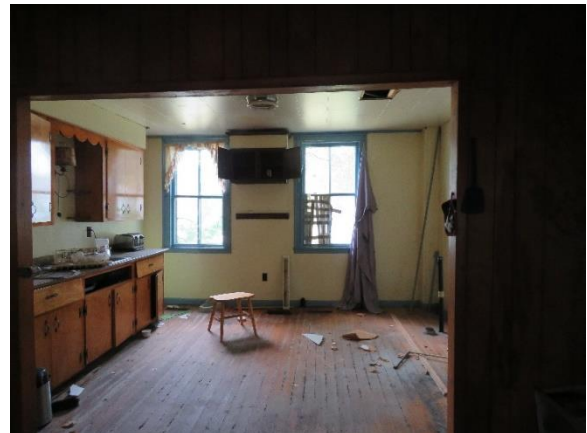
Figure 39 Main Building First Floor NE Room Looking North
