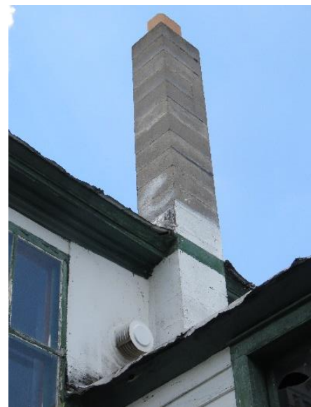
Figure 5 Concrete Block Chimney
