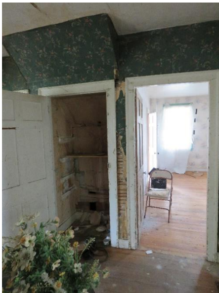
Figure 42 Main Building First Floor Center East Room Looking West
