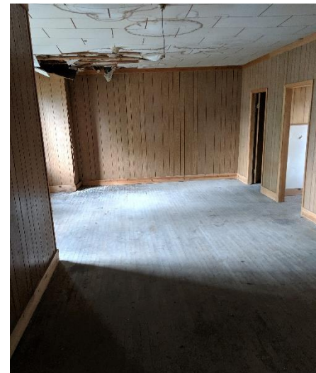
Figure 52 Ell First Floor Apartment
