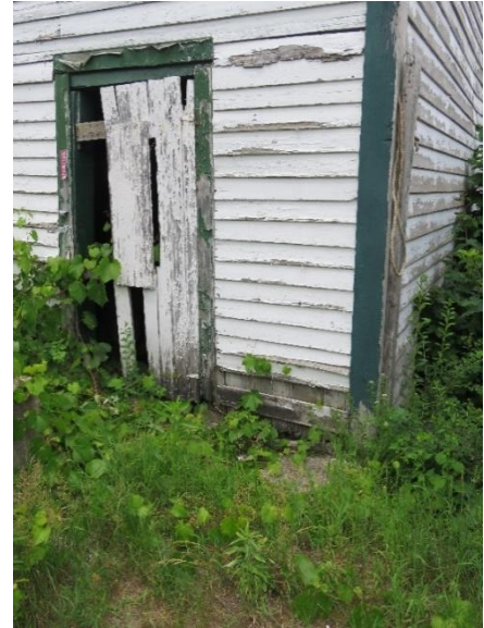
Figure 25 South Door to Storage
