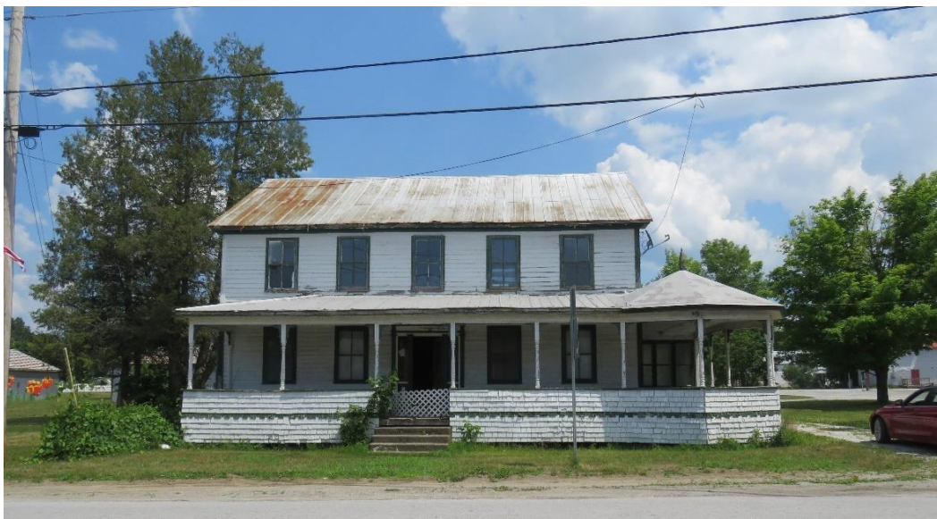
Figure 1 Exterior View Looking East
