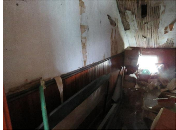
Figure 60 Ell Second Floor Room Looking North
