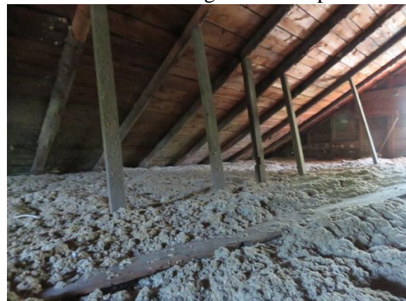
Figure 19 Roof Framing at Main Building
