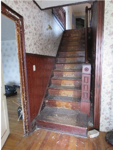
Figure 32 Entry Hall at Main Building
