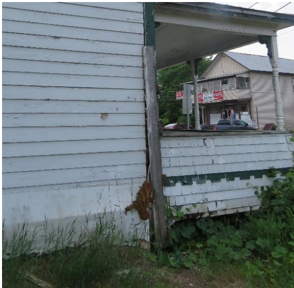
Figure 8 Vertical Corner Board at NW Corner
