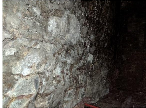
Figure 4 Stone Foundation
