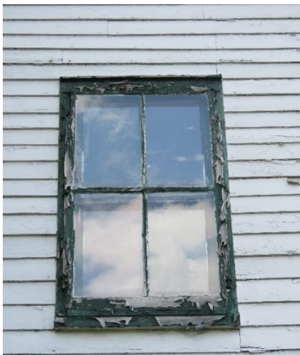
Figure 26 Typical Window at Main Building
