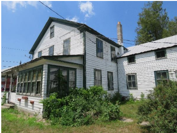
Figure 2 Exterior View Looking Northwest
