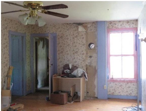
Figure 44 Main Building Second Floor Common Room Looking East
