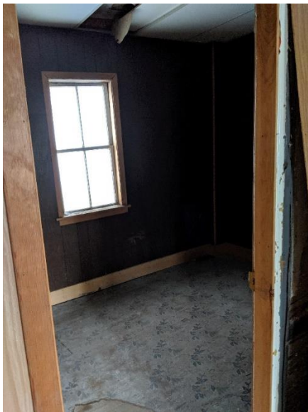
Figure 54 Ell First Floor Apartment Center North Room
