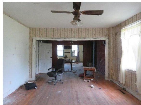
Figure 37 Main Building First Floor SE Room Looking North
