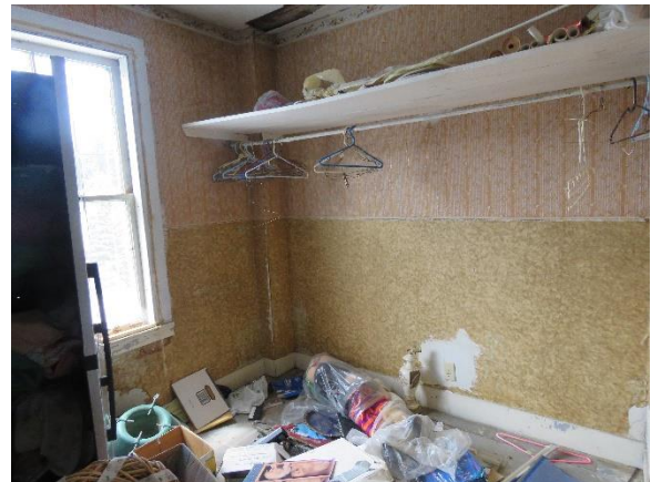
Figure 48 Main Building Second Floor Center West Room
