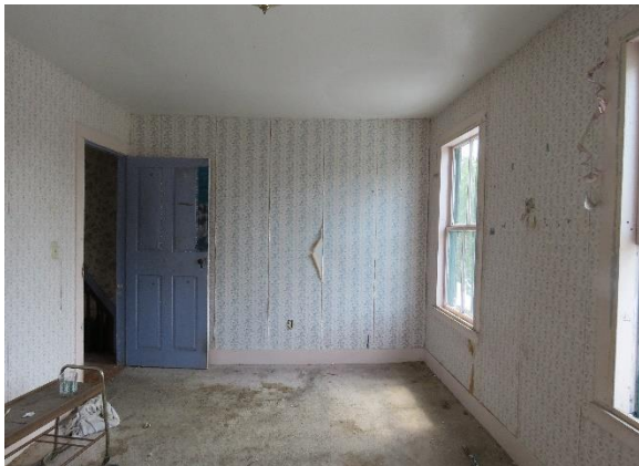
Figure 49 Main Building Second Floor NW Corner Room
