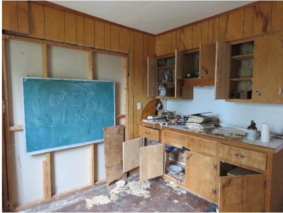
Figure 47 Main Building Second Floor Center South Room
