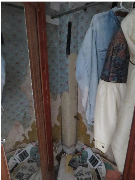
Figure 34 Wall Paper at First Floor NW Room
