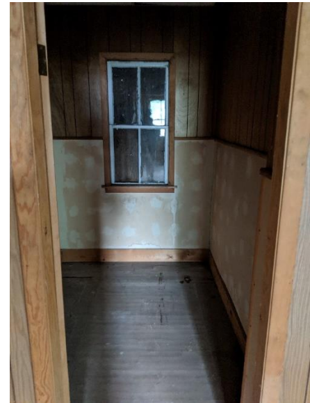
Figure 56 Ell First Floor Apartment NW Corner Room
