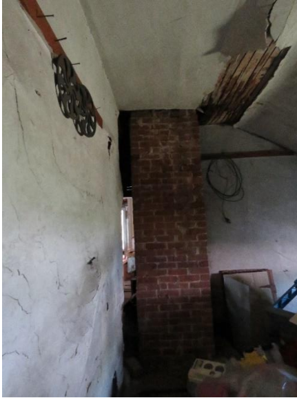
Figure 59 Ell Second Floor Room Looking West
