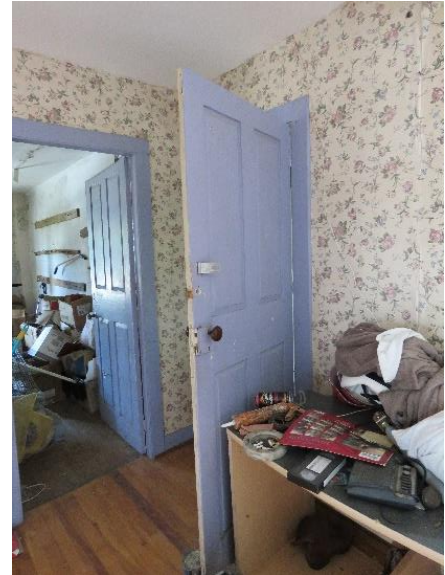
Figure 29 Main Building Second Floor Doors
