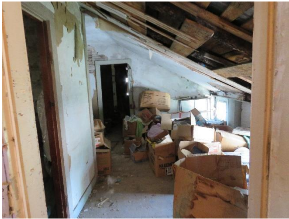
Figure 57 Ell Second Floor SW Corner Room Looking East
