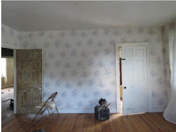
Figure 28 Main Building Northwest Room at First Floor
