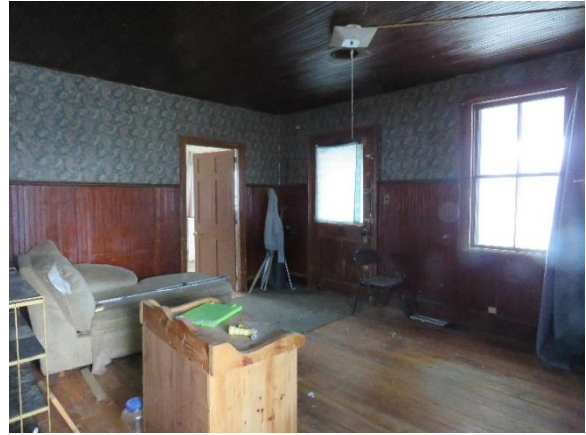
Figure 35 Main Building First Floor SW Room Looking Southeast
