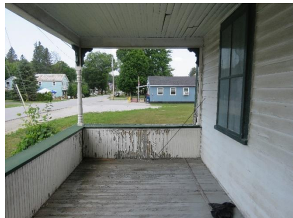
Figure 13 Porch Corner Looking North
