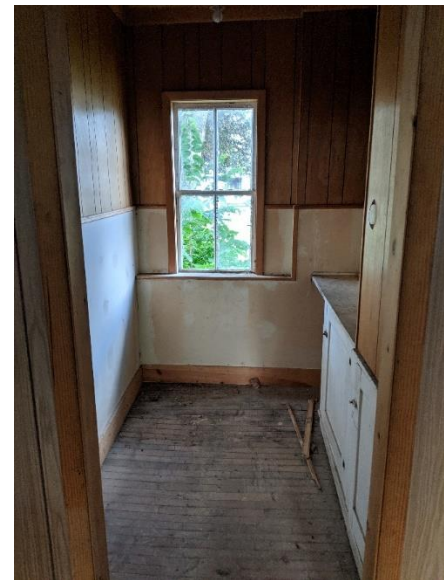
Figure 55 Ell First Floor Apartment Pantry
