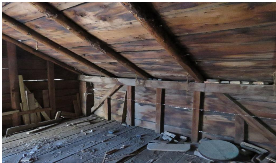
Figure 61 Ell Second Floor East Unfinished Cold Storage
