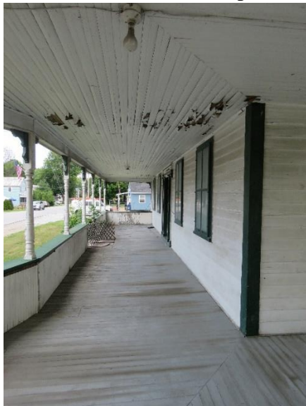
Figure 14 Porch Looking North
