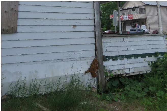
Figure 3 Foundation at Northwest Corner
