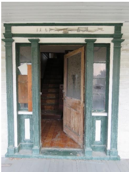
Figure 22 Entry to Main Building
