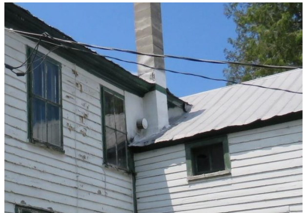
Figure 21 Roof at Main Building and Ell Intersection
