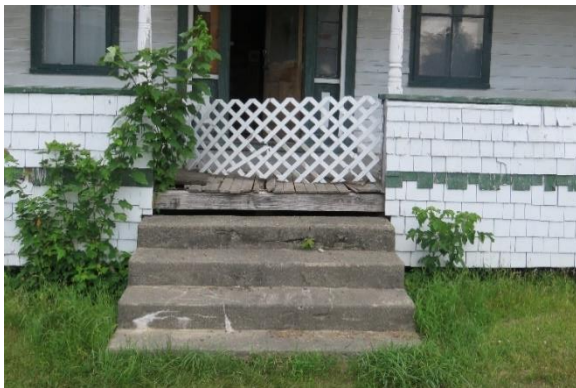
Figure 16 Porch Steps on West Side of Porch
