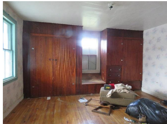
Figure 33 Main Building First Floor NW Room
