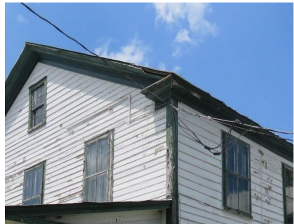
Figure 10 Cornice Return at Southeast Corner
