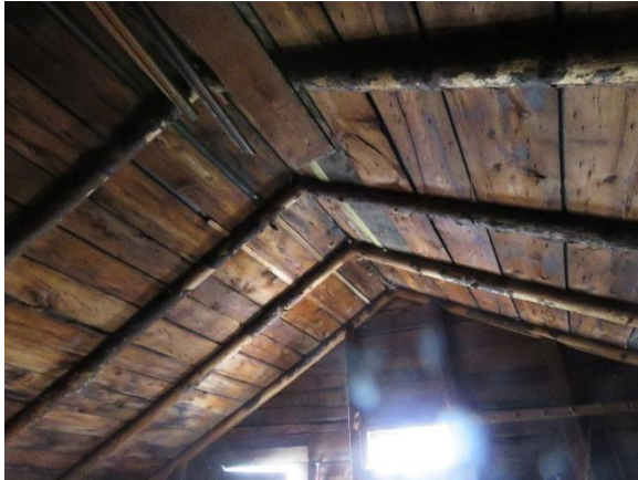
Figure 20 Roof Framing at Ell
